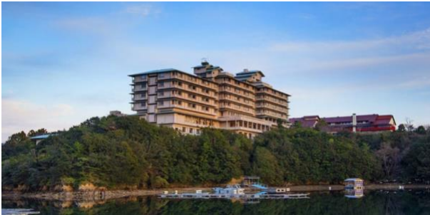
Building: Shima Kanko Hotel
